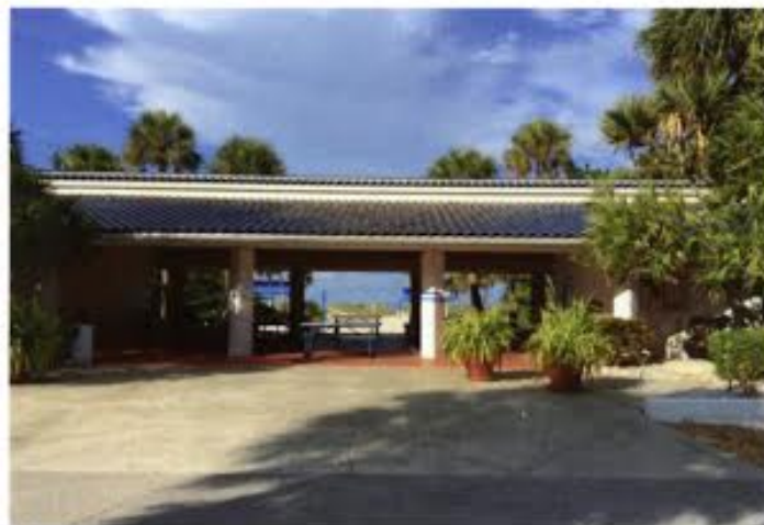
Completed Blue Tile
