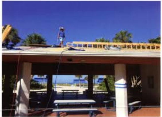
Construction of Vent System on Roof
