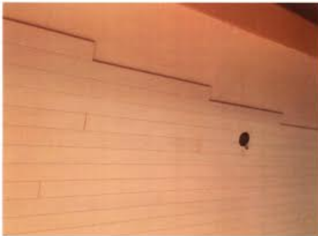
Installation of Wood Siding on Ceiling of Pavilion
